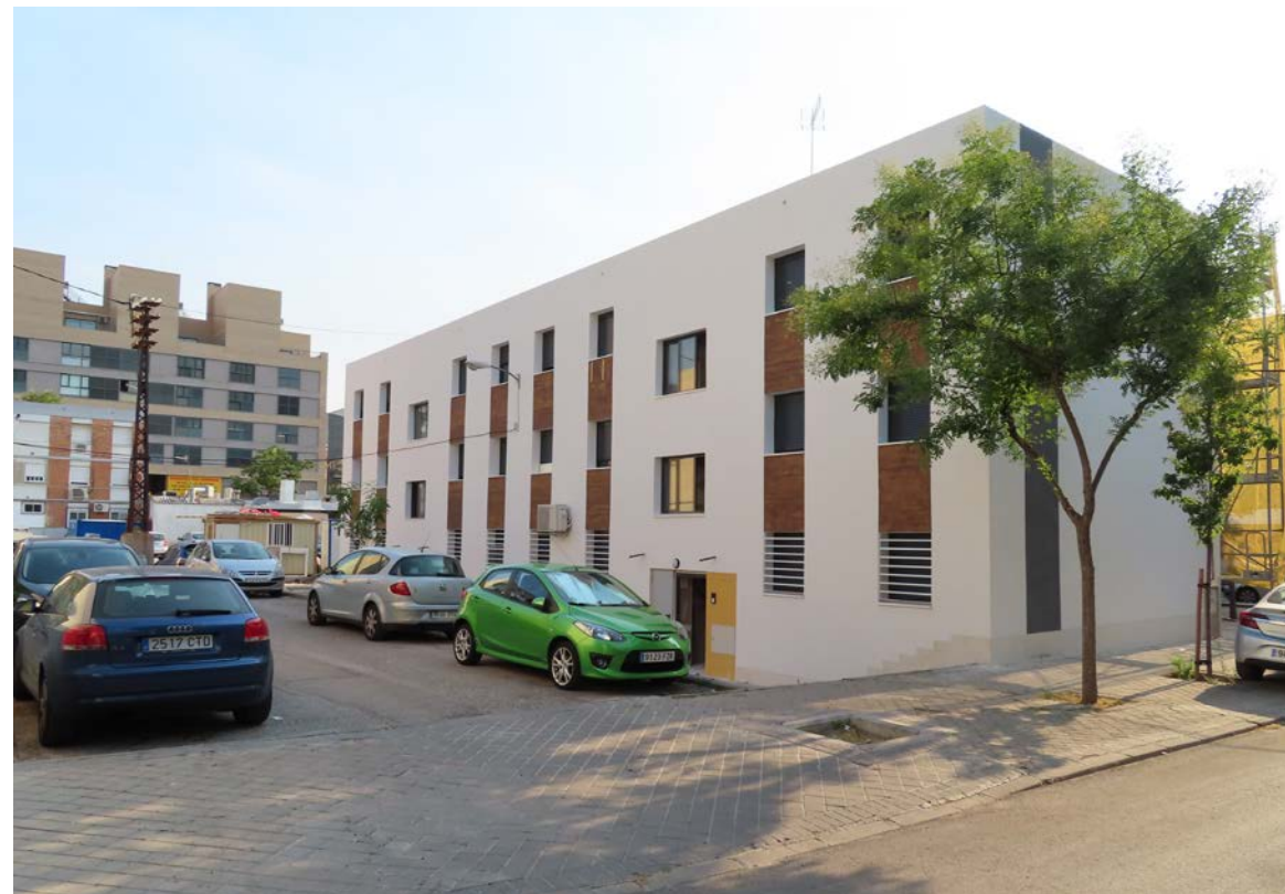
Same building AFTER rehabilitation
